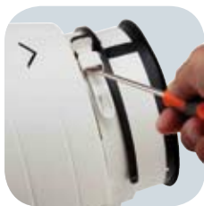
Loosen and open clamps on both sides
