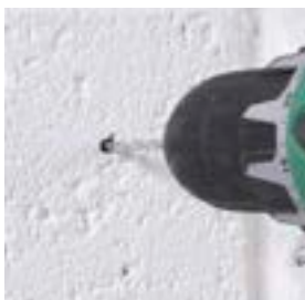
Drill a 5mm pilot hole
