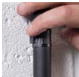
Secure cable with locking tab
